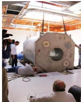
That meant creating a slab independent of the building foundation and on separate footings. "It's kind of a standalone pedestal that the magnet sits on," he says.
